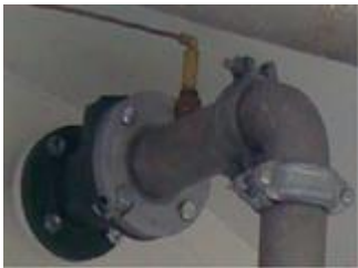
EASY TO INSTALL USING WITH A 1/4" FLEX CONNECTOR OR 1/4" TUBING INTO THE PRODUCT PIPE
